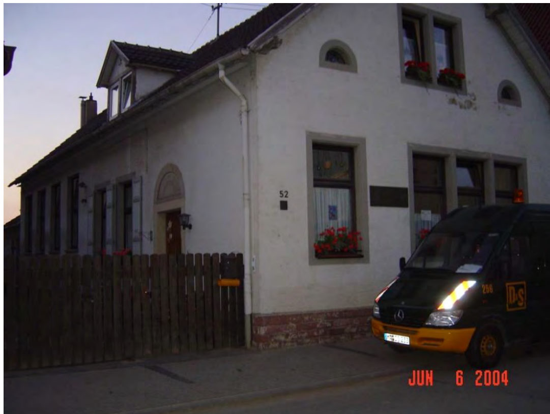
Above the entry door is the lintel.
